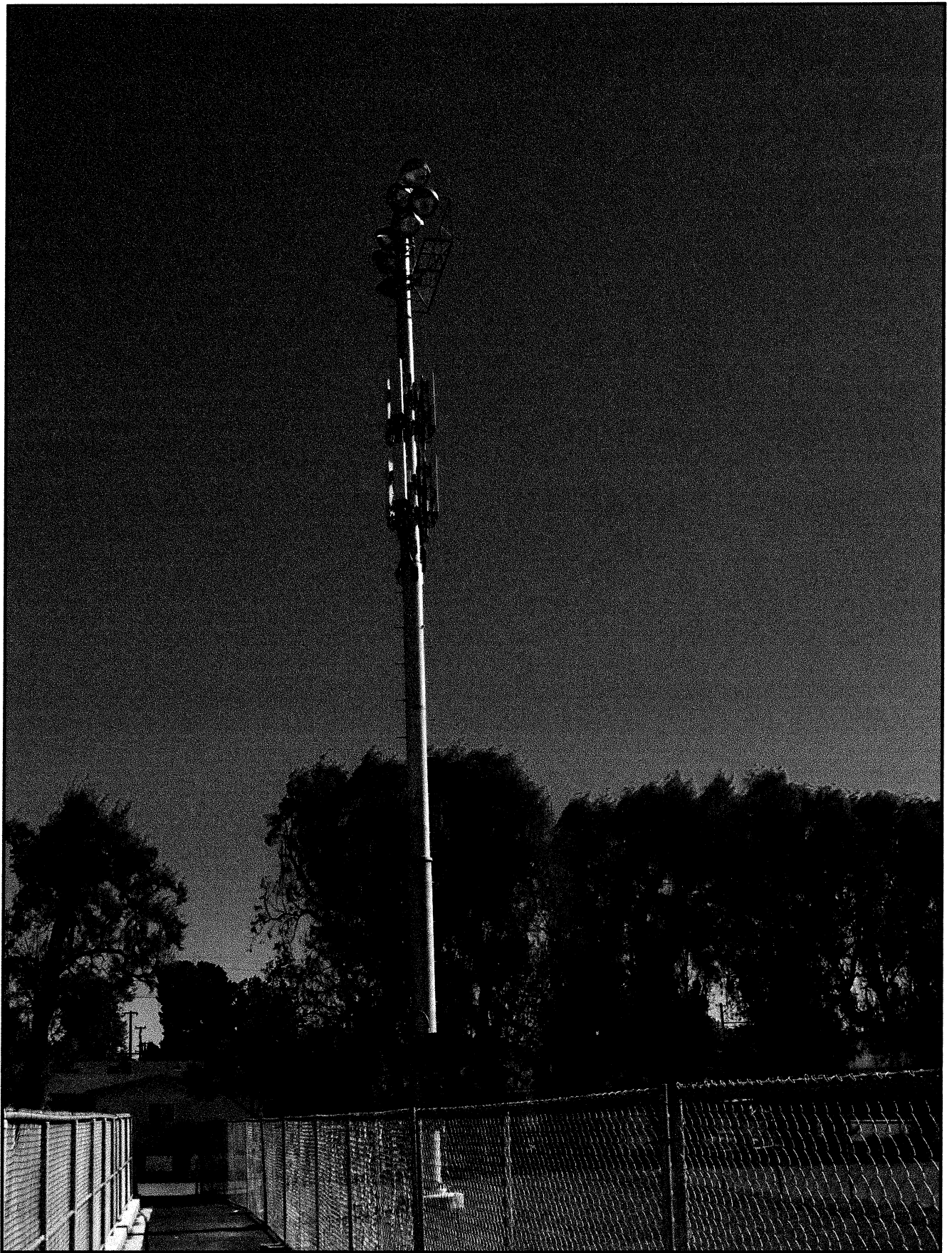
Pleasant Valley Park in Camarillo (Underground Vault)
